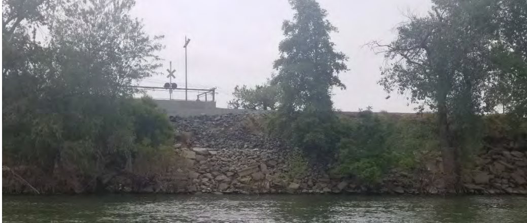
Figure 2-3 - RM 58.65 is at the downstream end of the Old Sacramento River floodwall where a variety of rip rap, cobble and broken concrete has been placed over the erosion and slumping that has occurred.
