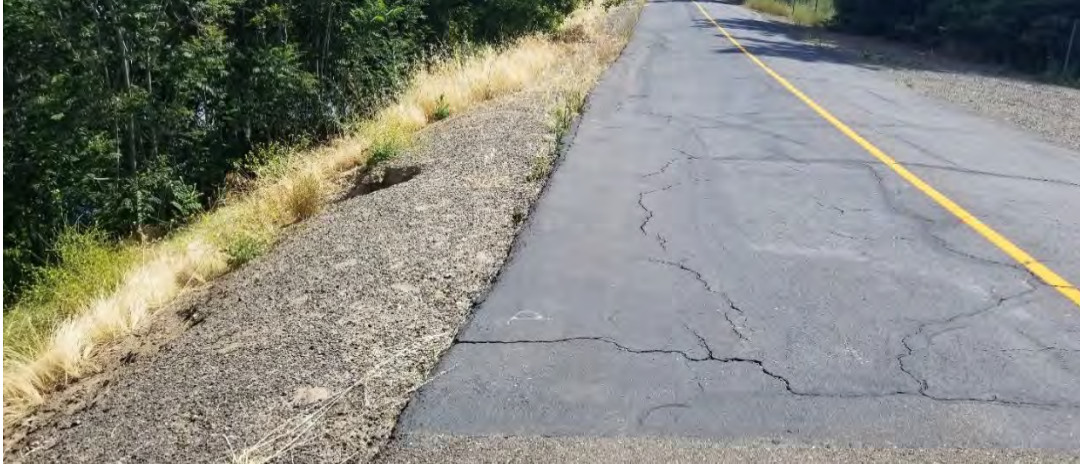
Figure 2-7 - RM 55.55 looking upstream at levee top near the Westin Hotel parking lot showing tension cracks, possibly indicative of landslide headcut and evidence of past repairs to the bike path on the waterside levee slope. This location has no berm and the waterside levee face extends into the left bank of the river.
