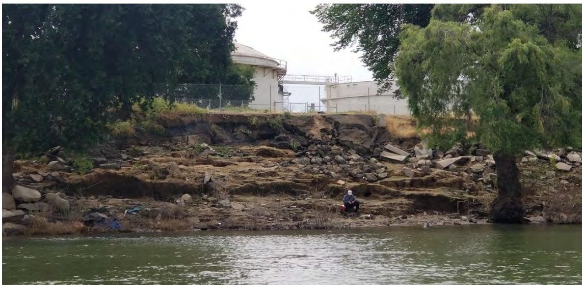
Figure 2-5 - RM 58.2 North of Miller Park and Marina where concrete and asphalt waste rubble has been placed ongoing erosion is evidenced by the crumbling asphalt road and slumping bank slope.
