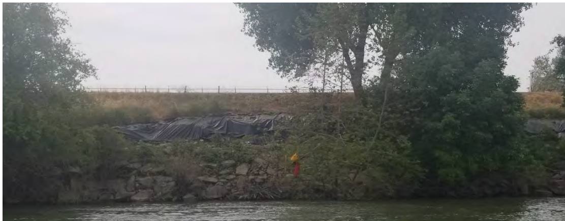
Figure 2-4 - RM 58.45 is located at the Pioneer Reservoir. Recent erosion behind existing rock and concrete rubble has prompted emergency repairs with black plastic sheeting.
