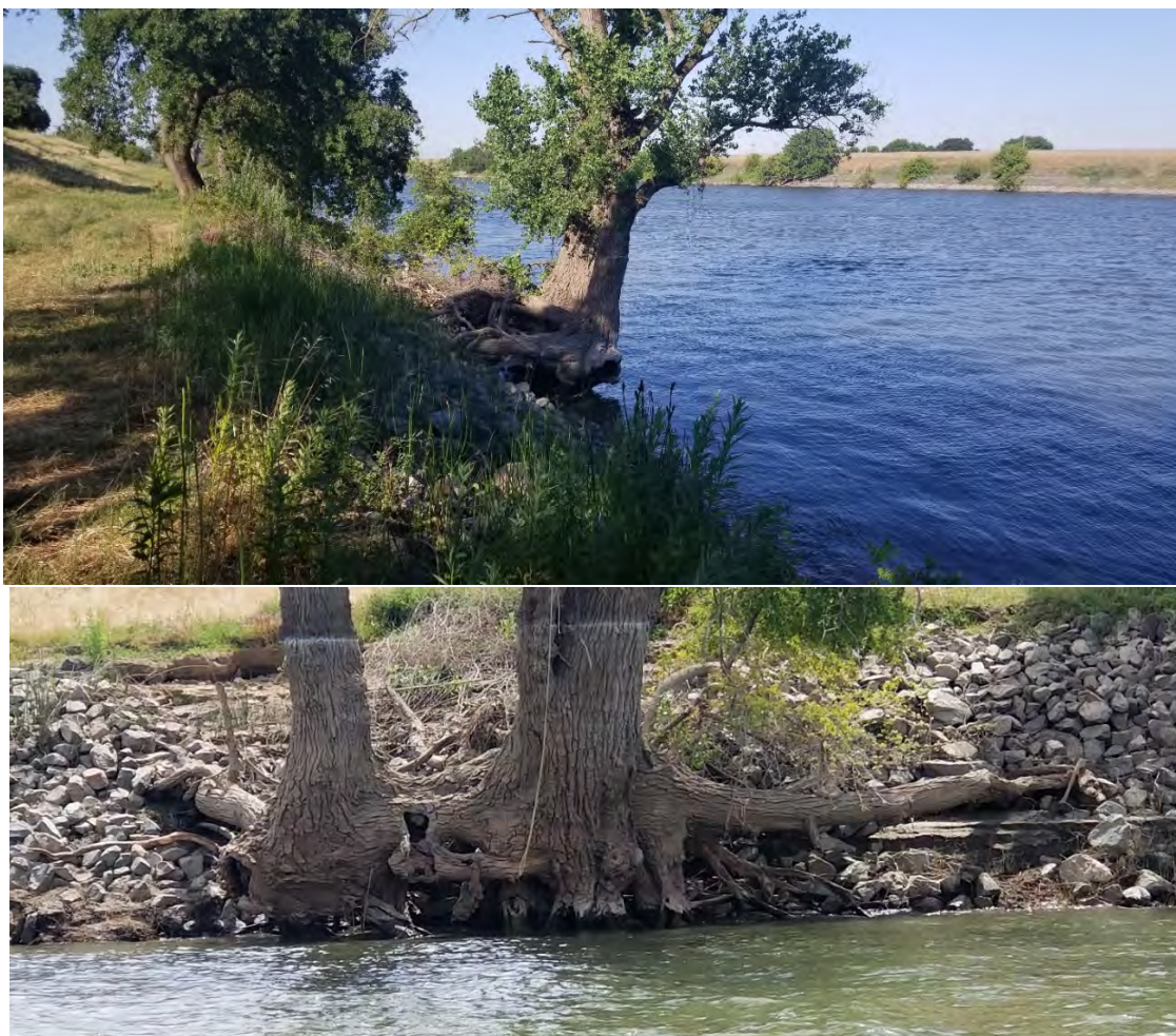
Figure 2-9a and 2-9b – Land and waterside views at RM 51.9 at the north-west corner of the Pocket area has shows extreme erosion around tree roots, a narrow berm and spot repair rip rap.
