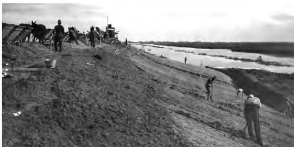
The Lisbon Levee in the Yolo Basin, part of Reclamation District 307, receives a concrete facing in 1911. The four inch thick concrete, reinforced by a wire mesh, was the first such large scale application to a river levee, covering two and a half miles.
