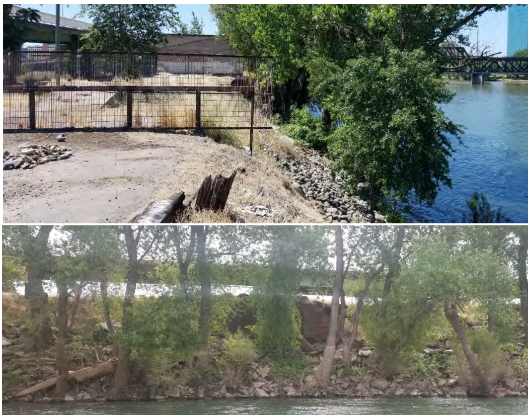
Figure 2-2a and 2-2b - RM 59.55 Land and Waterside Views of Bank Located Near the I St Gage and the I St Bridge with an Abandoned Building, Power Poles, Older Rip Rap, Cobble and Rubble Line a Slumping Bank.
