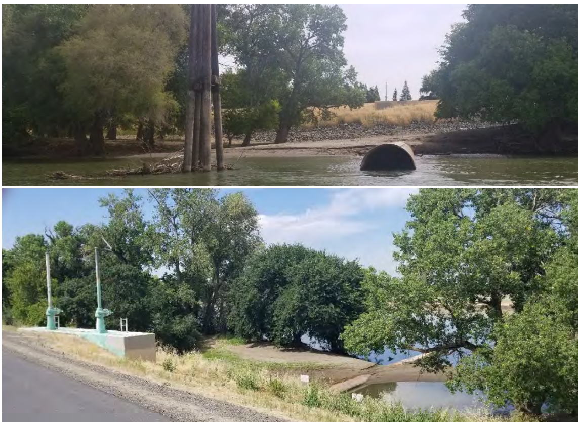
Figure 2-6a and 2-6 b - RM 56.5 Views from boat (top) and levee top (bottom) of erosion around storm drain outlet.
